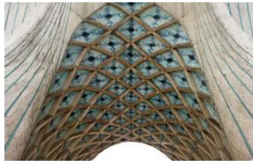
3: Above the arch of the Sassanid there is a half zigzag arc that is repeated in north-south side also.
