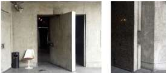
10: The central stone doors (in imitation of Persepolis)
